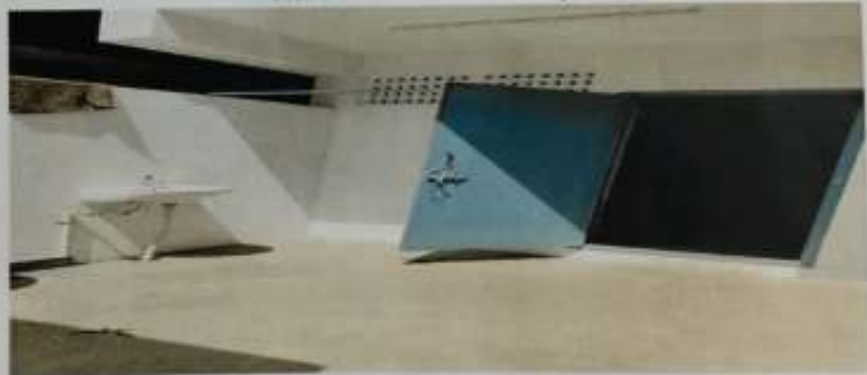
Women's Wash Rooms: Behind Food Court
